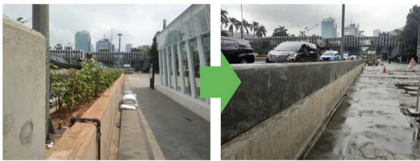
Penambahan Dinding Penahan Air Limpasan (21 Jan 2020)
