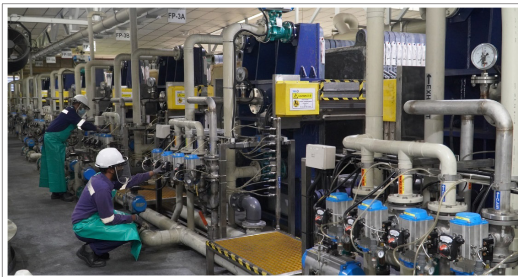
[Figure 4-8] Powder Processing Equipment
