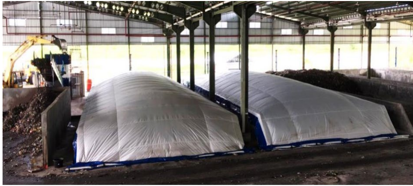
Gambar 3.7 Bio-drying di fasilitas RDF Plant Cilacap
